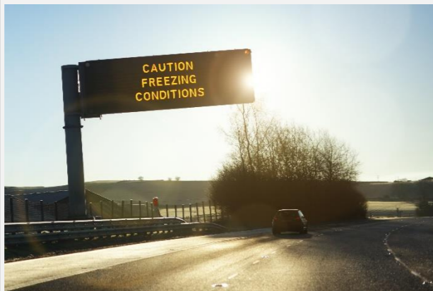
Figure 4-16: Cantilever VMS sign
