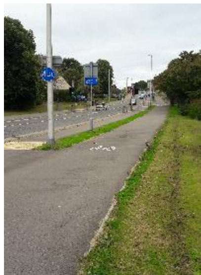
Photo 5 - Segregated section on Tillydrone Road
